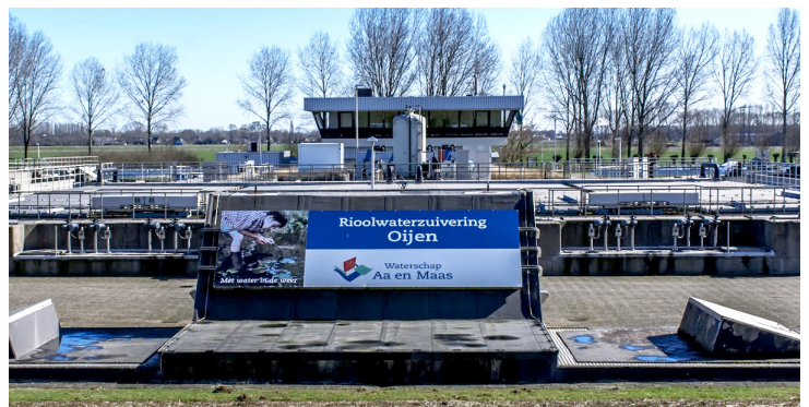
The Oijen WWTP serves a population of approximately 350,000
